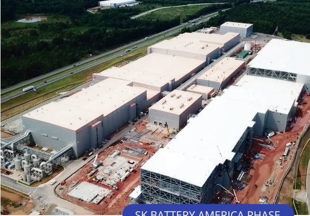
SK BATTERY AMERICA PHASE
